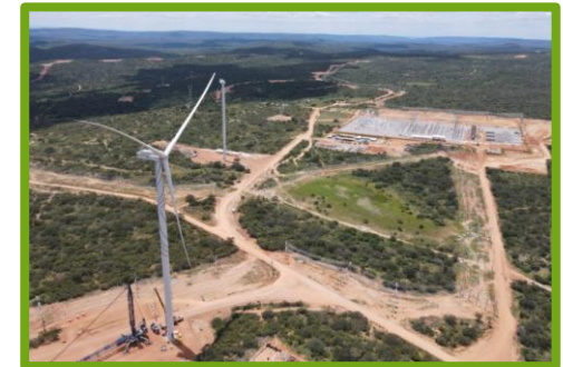
PHOTO: Assembly of OITIS 5 wind turbine with SE in the background
