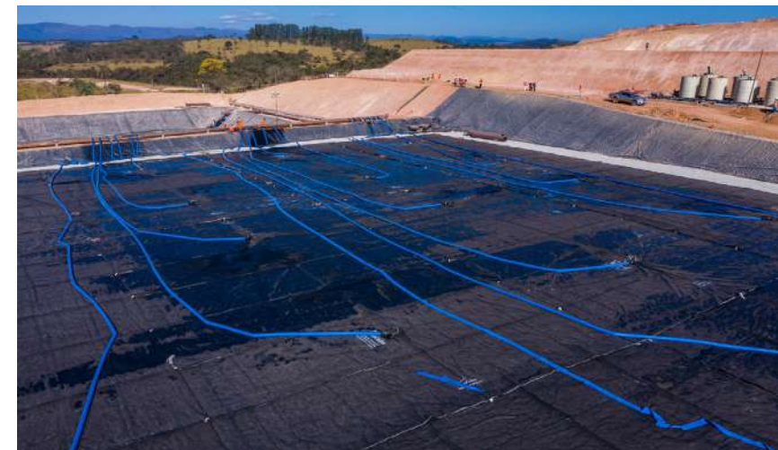
Overview of bags used for storage and dehydration of tailings dredging. The water drained from these bags is pumped to ETAF and returns clean to the Paraopeba river. Photo: Vale Archive.
