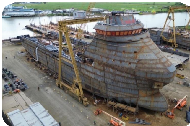
PSV 5,500, with delivery expected in June 2026, currently under construction at the Detroit shipyard in Itajaí, Santa Catarina
